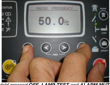
Hold pressed OFF, LAMP TEST and ALARM MUTE
